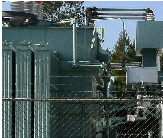
Transformer with Reactor Grounding System
